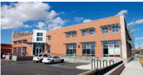
Top: Loft space was created by using materials found in the abandoned building. Above: Shading devices above every window significantly decrease interior heat gain.
