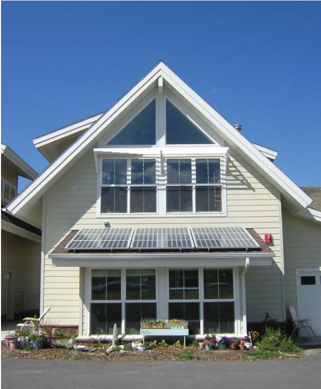
Left: Photovoltaic array above the sunspaces. Top: The steep site permitted daylighting of the lower level. Above: Interior view of residence. © Erik Hendrickson/National Park Service
