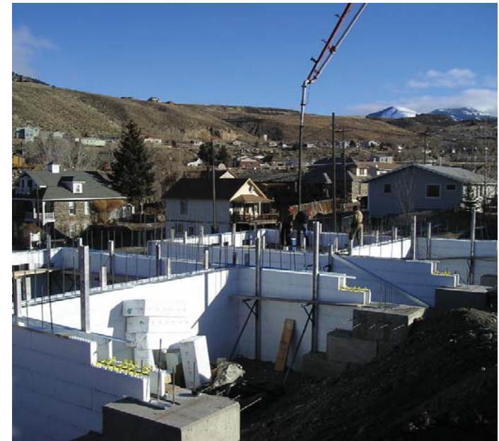
Shown during construction, the Insulated Concrete Form (ICF) system was used for both foundations and walls in order to stabilize heat transfer. © Erik Hendrickson/National Park Service
