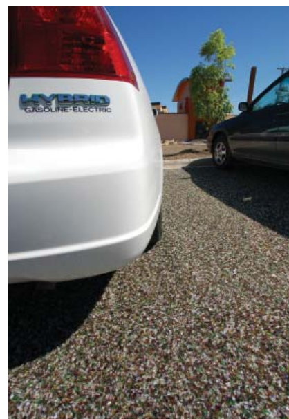
A 10-kilowatt photovoltaic array generates approximately 35 percent of the building's annual energy needs. Near Right: Permeable pavement employing recycled glass cullet reduces the urban heat-island effect, recharges the aquifer, and eliminates pollution to waterways. Far Right: Light shelves direct natural light deep into the interior. Artificial lighting is not required in most rooms during daylight hours.
