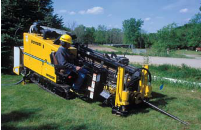
Pella, Iowa has a robust manufacturing industry cluster, with companies that manufacture equipment such as the directional boring equipment seen here. Manufacturing jobs account for 60% of all labor income in Marion County, Iowa, where Pella is located. Photo courtesy of PADCO.
