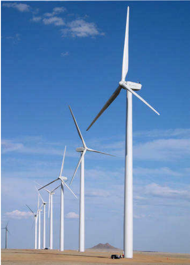
At the time of its construction in Prowers County, the Colorado Green Wind Energy Project, which has 108 1.5 MW wind turbines was the largest wind farm in Colorado and one of the largest in the country. Photo courtesy of Prowers County Economic Development, Inc.
